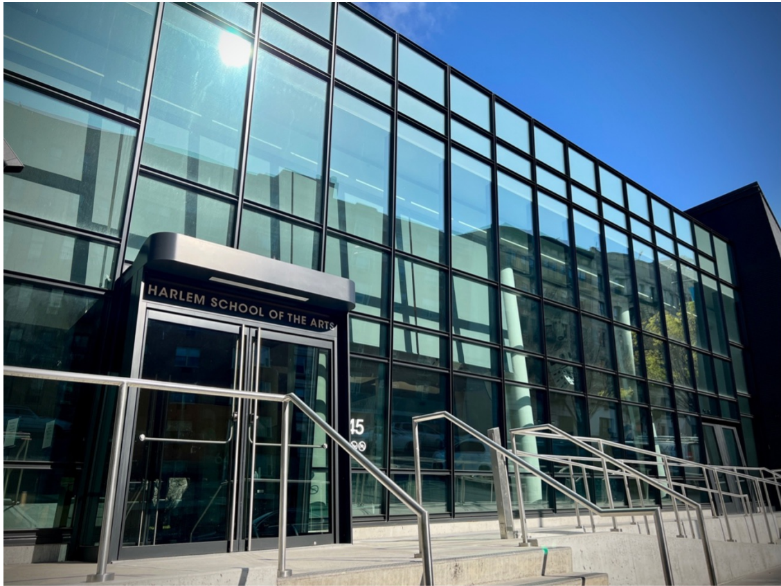
While much of the city sat dormant during the early days of the pandemic, a $9.5M renovation project was happening at the Harlem School for the Arts, located on St. Nicholas Avenue in Harlem. Photo by Gary Hilborn.
